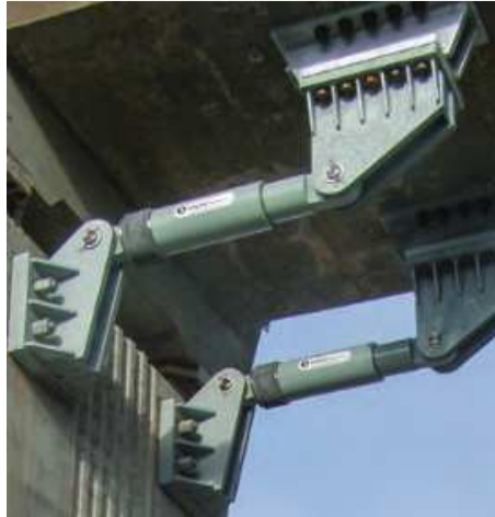
Figura 19 - Sistema de controle de sismos (Seattle Central Light Rail, Seattle, EUA) (Taylor Devices).
