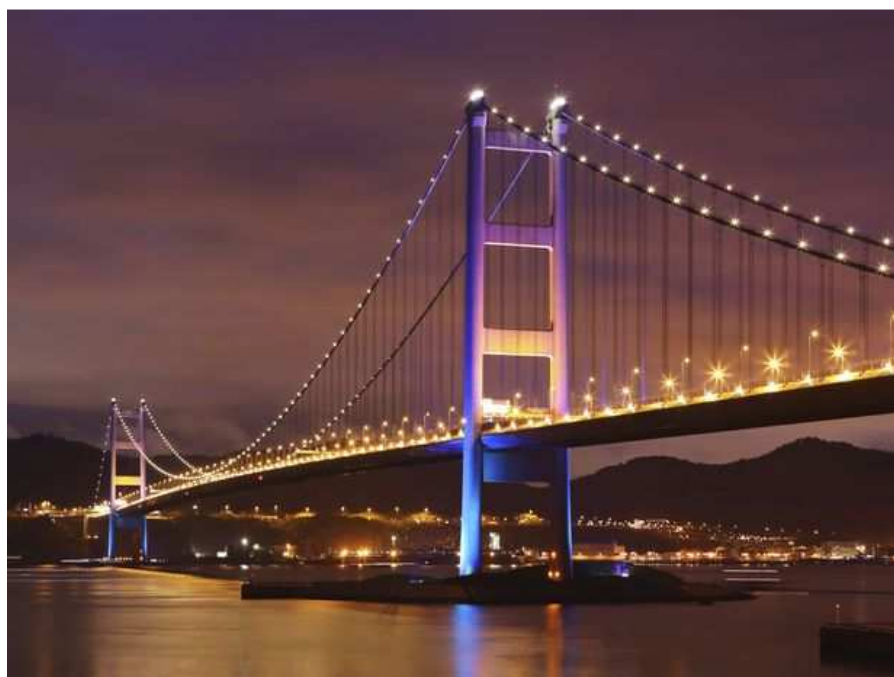
Figura 1 – Ponte Tsing Ma – Hong Kong [1].
