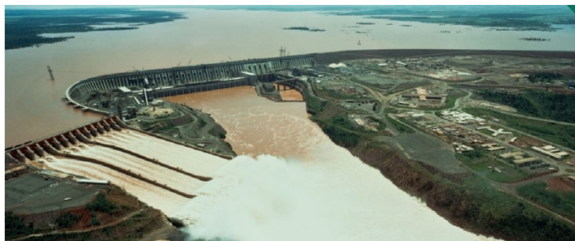
Figure 1 – Lake and reservoir view of Itaipu hydroelectric plant
