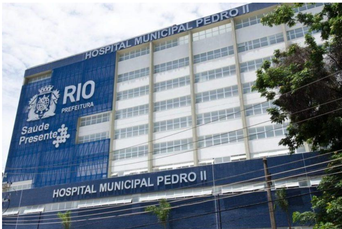
Figura 11 – Hospital Municipal Pedro II.
