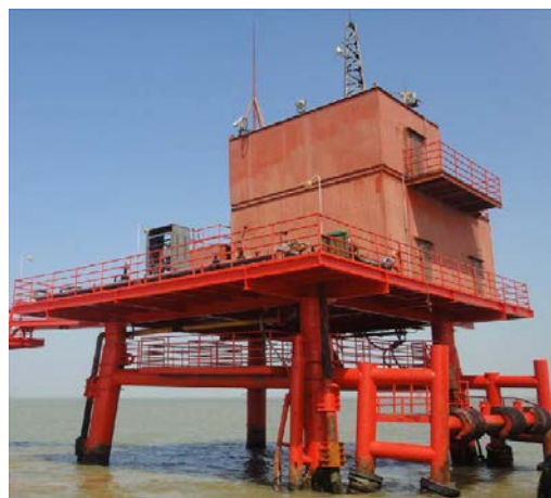
Figure 2 - CFDST columns used in an offshore platform [5].
