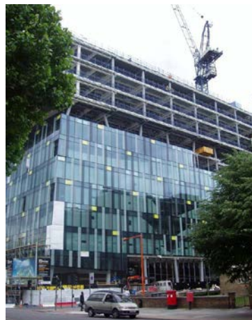
Figure 5 - CFDST columns in a high-rise building, Office Building Palestra, London [13].
