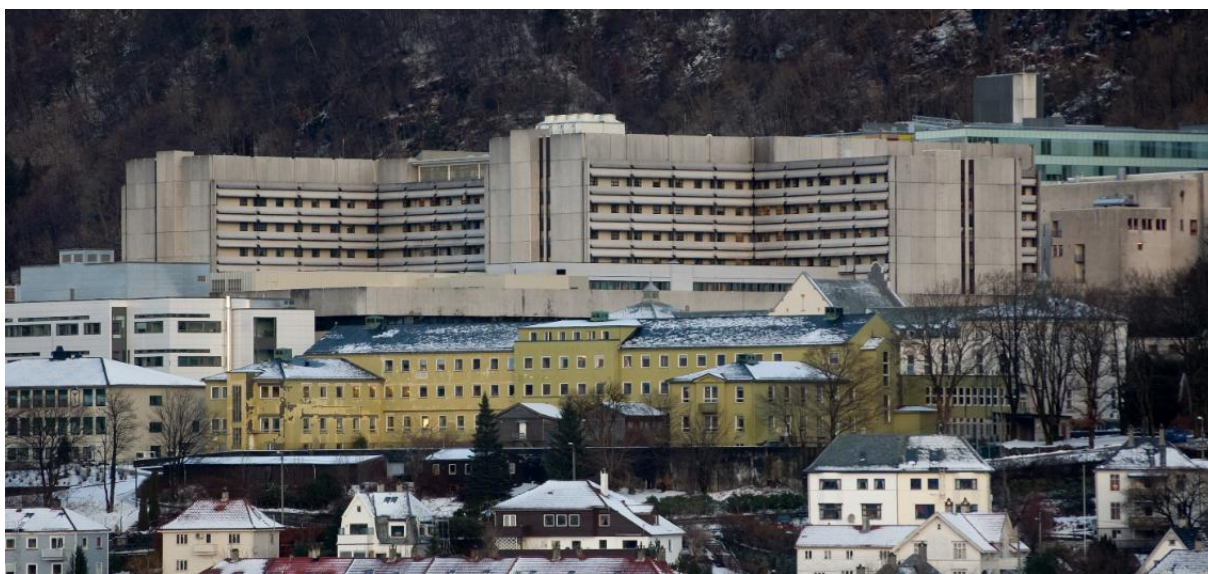
Figura 1 – Haukeland Hospital – Bergen - Noruega
